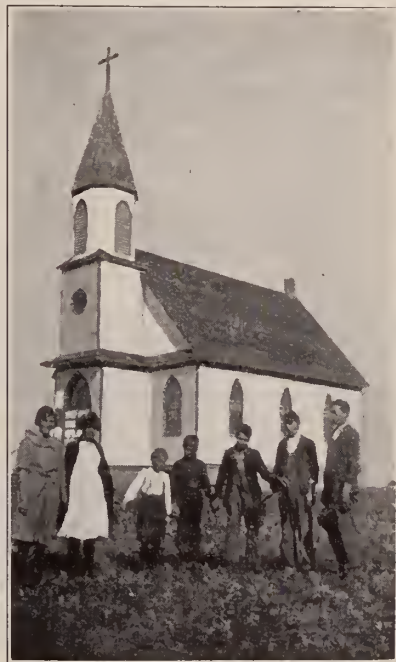
MARTIN'S REFORMED CHURCH, VECREVILLE, ALBERTA, CANADA.
